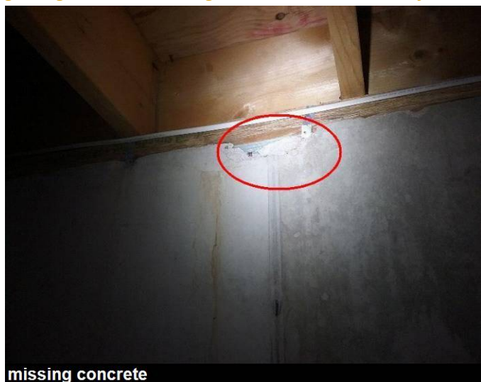
right side basement - settlement crack
